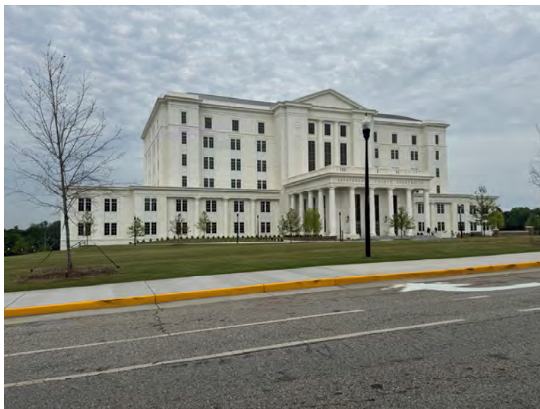
Site Visit at Tindall Corporation and Photo of a Building Casted with the New Architectural Mix
