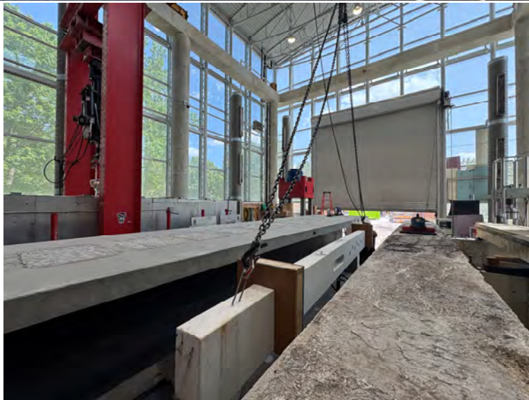
Lifting and Big Beam Transported to CFL
