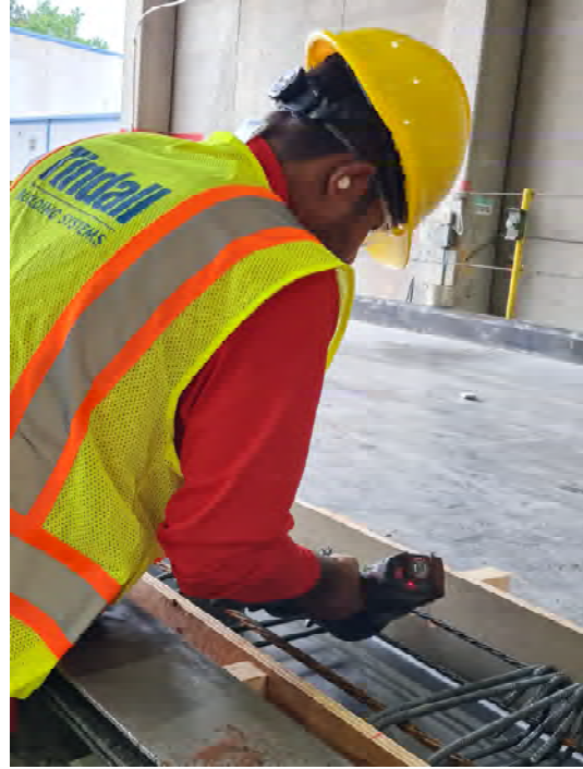
Building the Formwork and Placing Reinforcement
