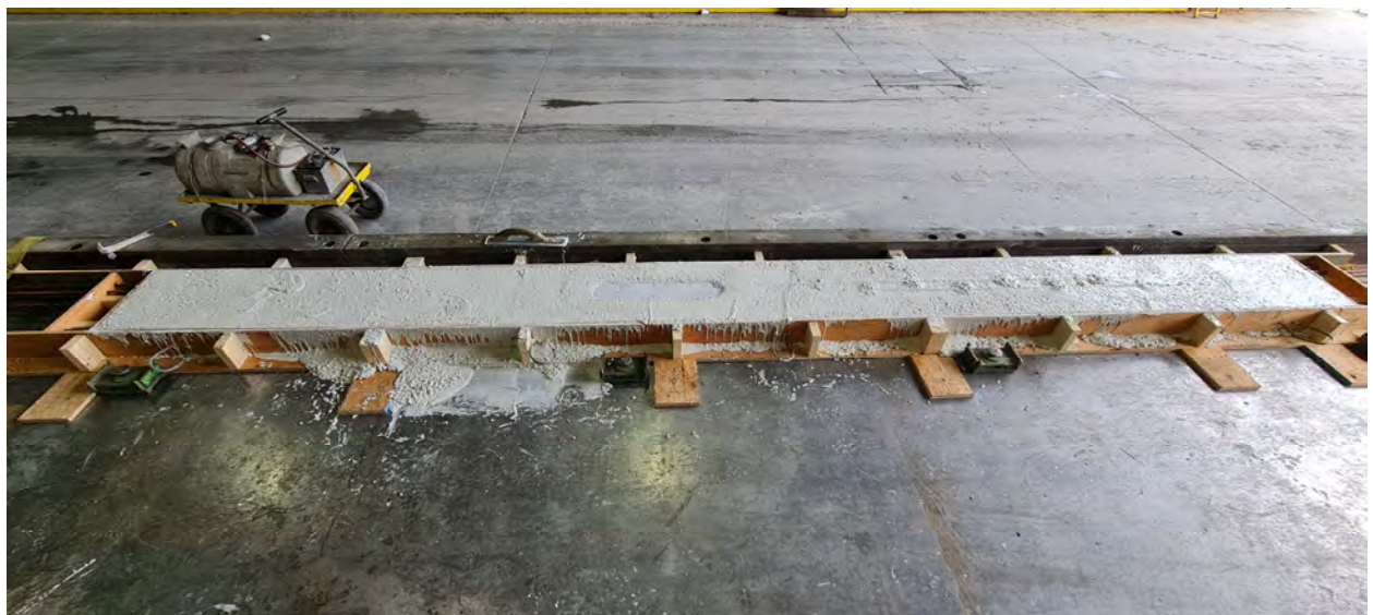
Batching of Concrete Mix and Casting at Site
