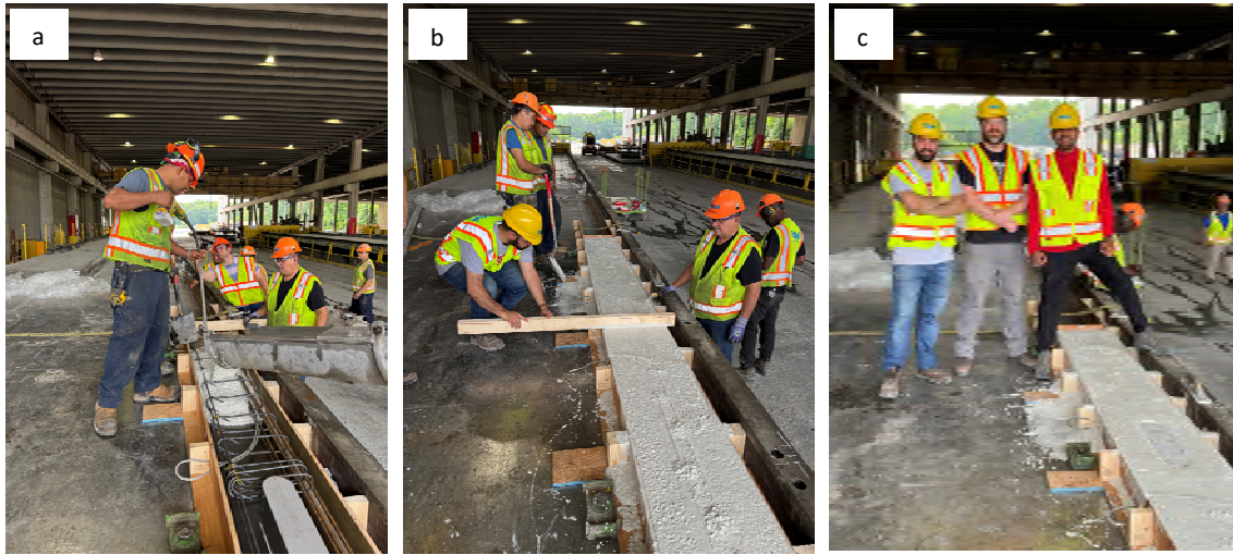
Figure 16: Casting the Big Beam using an architectural mix
