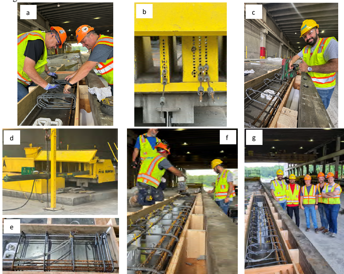
Figure 15: Placing reinforcement within the formwork
